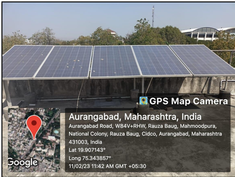
Photograph Showing Installed Solar Panel at Institute Roof
